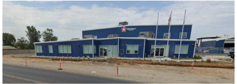
Figure 48. Republic Services Fresno local office.
