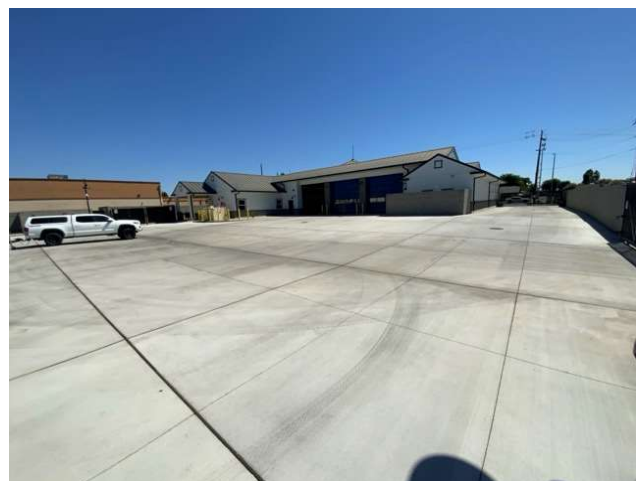
18 - REAR PARKING LOT
