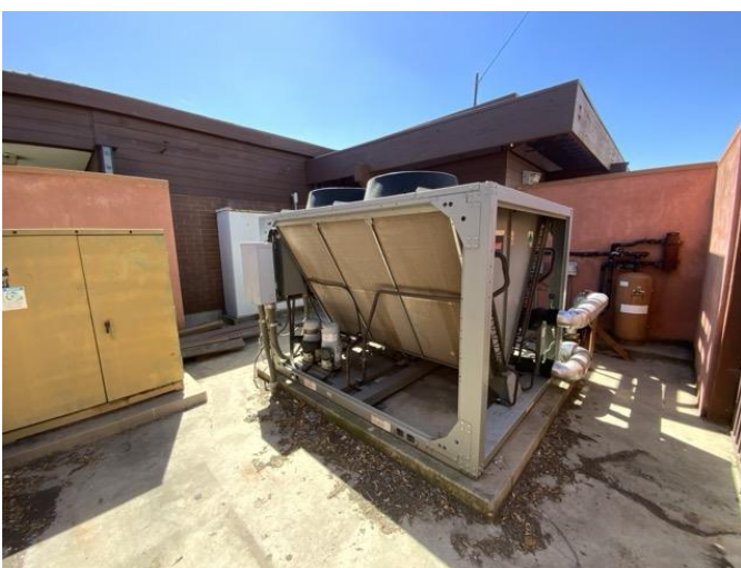
17 - EXTERIOR MECHANICAL SPACE
