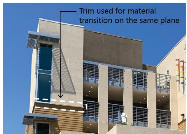
Example trim used to transition between exterior building materials.
