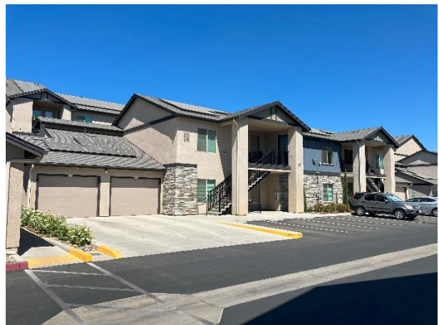
Driveway apron in front of garage door
