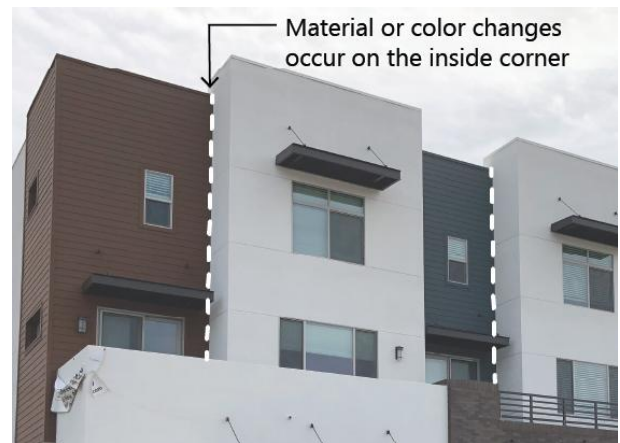
Example of changes in exterior finish material on the inside corner of a building.
