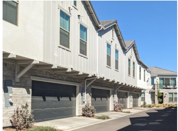
Example of gutters, downspouts, and trim being of a consistent color.
