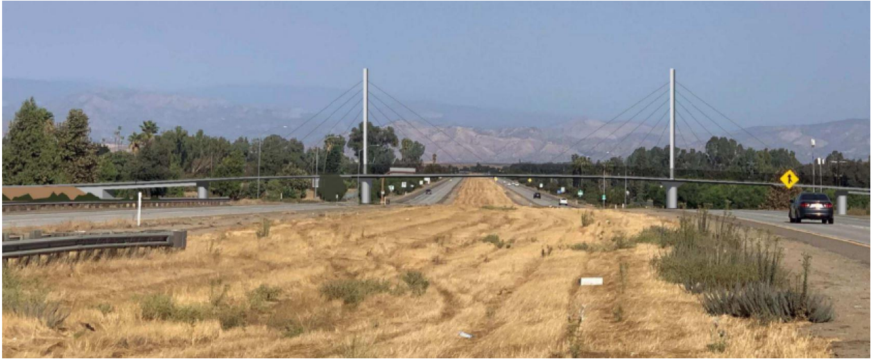
Figure 4 – Signature Cable-Stayed Bridge: $36.8M Total Cost
