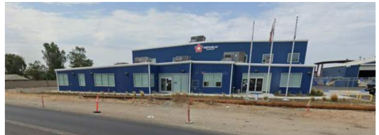
Figure 48. Republic Services Fresno local office.
